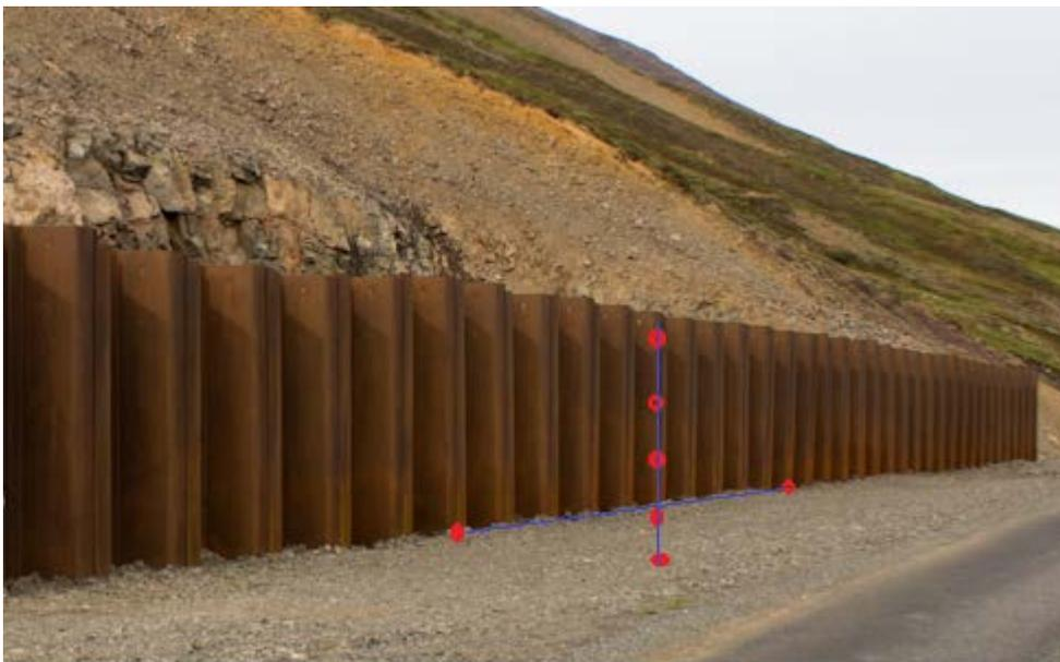
Figure 6. Red dots indicates the location of the strain gauges. The four dots seen on the ground indicate strain gauges in the ground.
