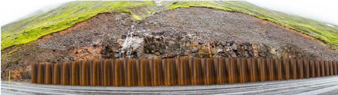
Figure 3. The sheet pile wall in avalanche path no 37.
