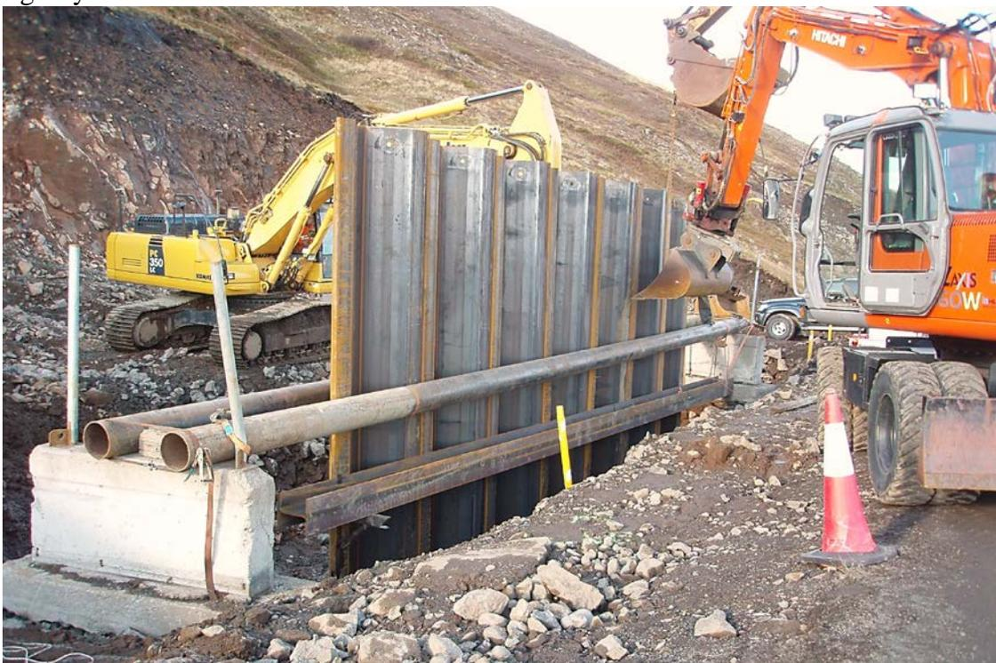
Figure 5. Installation of the steel sheet piles. Here the steel sheet piles are guided by steel pipes while the trench is filled with boulders and gravel. Photo: IRCA.
